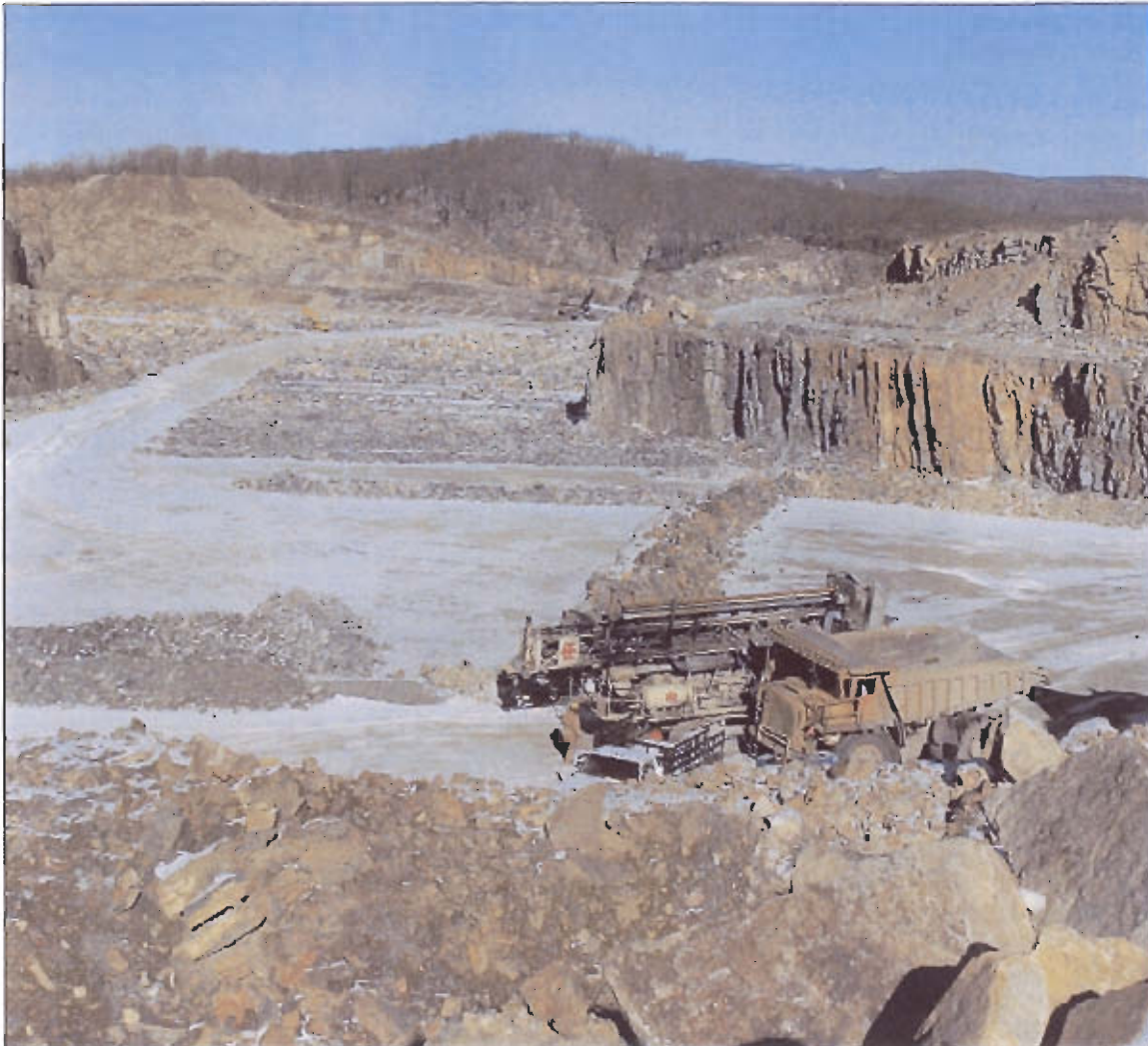
Tilcon New York's Pompton Lakes, NJ quarry (formerly Passaic Crushed Stone) is a 300-acre granite/gneiss rich site that yields better than 1.6 million tons of crushed stone product per year. The company has been at this same site since 1956 and primarily produces 3/4-inch, 3/8-inch, 1/4-inch products, as well as screenings.
