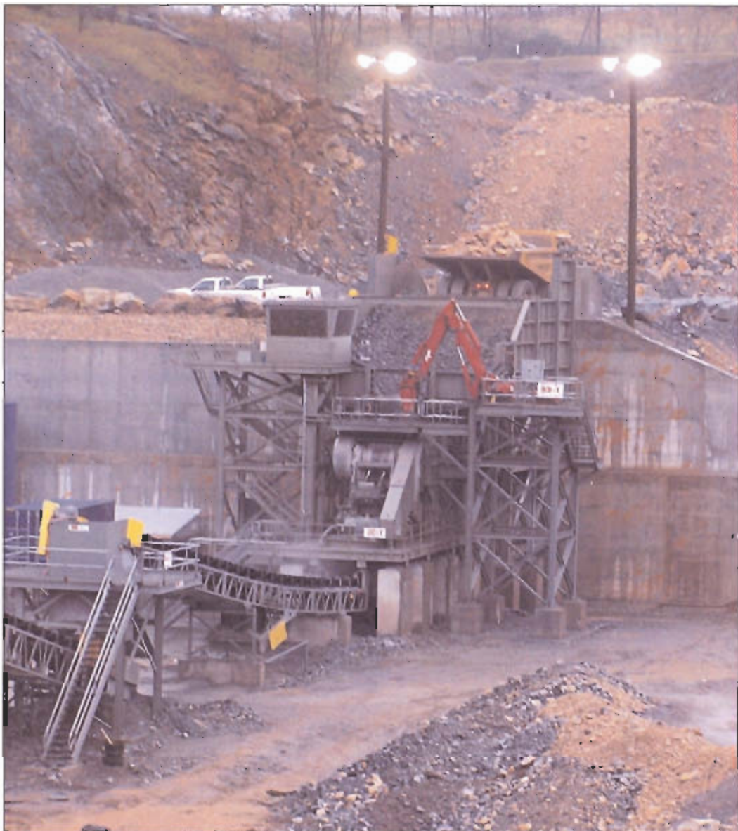
New TelSmith 4448 primary crusher installed at new plant.
